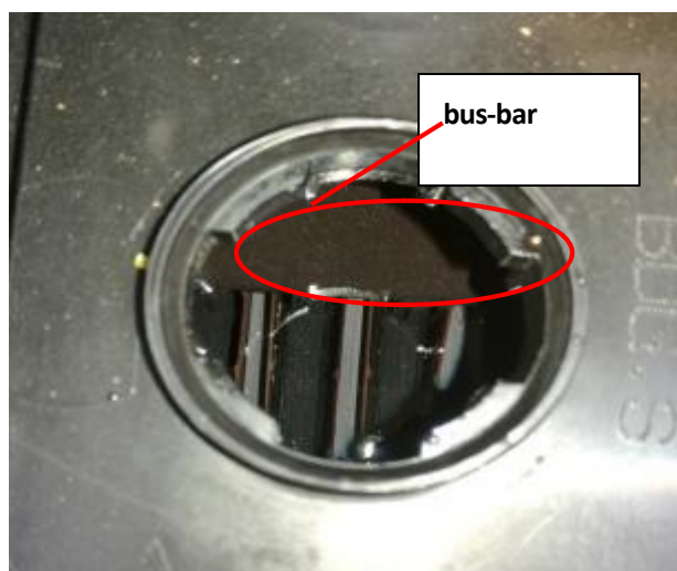
3. Electrolyte lever is lower than bus-bar, then add distill water
